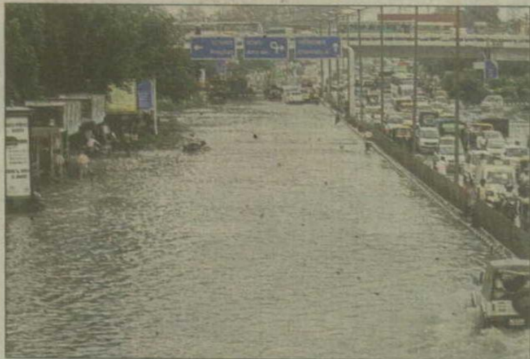
■ Improper drainage, water logging were the reasons behind 60% of traffic snarls in the period between April and September. HT FILE PHOTO
